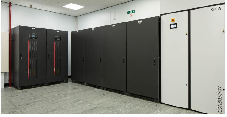
The final **modular data centre** design incorporated 20 cabinets, full power supply infrastructure including generator hook up, hot aisle capture configuration for energy efficiency, Novec Fire suppression and Wagner early particle detection to ensure safety as well as energy efficient air conditioning and UPS systems in an N+1 format and all 19" cabinets included intelligent power distribution.
