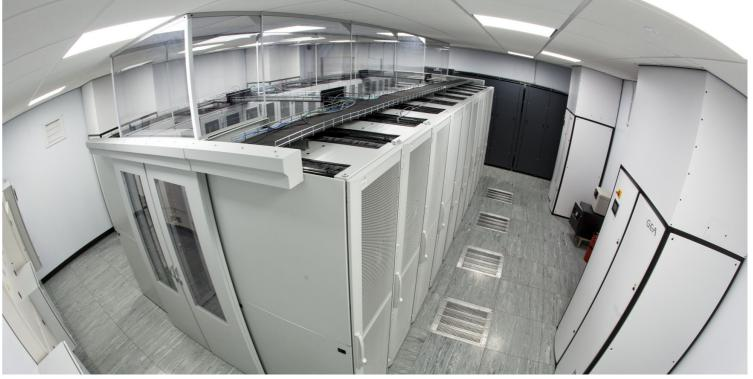
Equipment included an external modular room building to secure 20 x 19" cabinets, hot aisle capture, N+1 UPS, raised access flooring, Novec Fire suppression and VESDA detection and energy efficient LED lighting. Highly energy efficient air conditioning was installed with plug fan and EC motor technology allowing the systems to ramp up and down as the cooling requirement demands.
